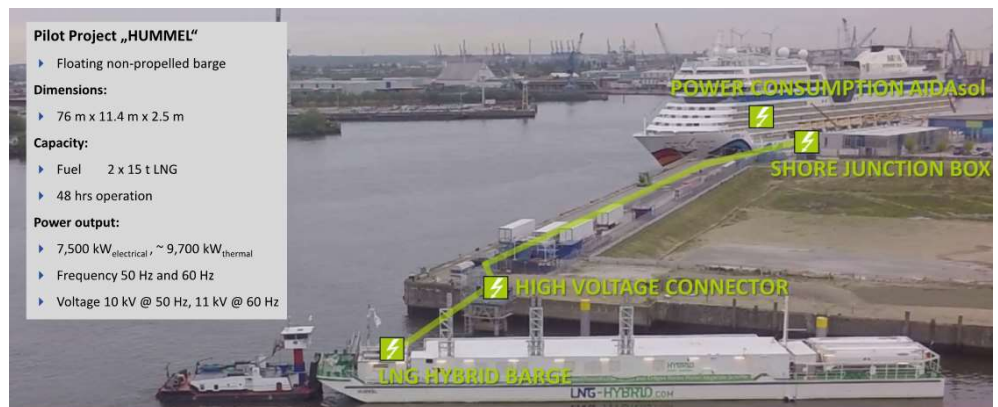
Figure 2: Illustration of LNG barge. The barge at the bottom of the photo is connected to the cruise ship by cables running along the quay and a junction box by the ship. Source: Hybrid Port Energy. Becker Marine Systems.
